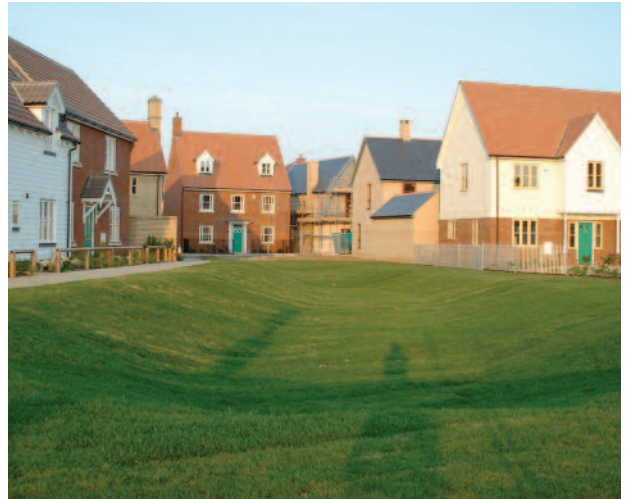
Infiltration basin in dry state, Ipswich
