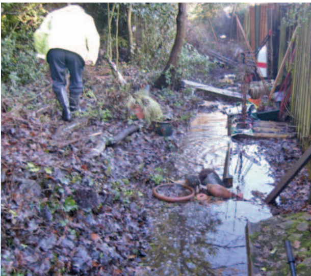
Figure 5.5: Watercourse blocked with debris, Ipswich
