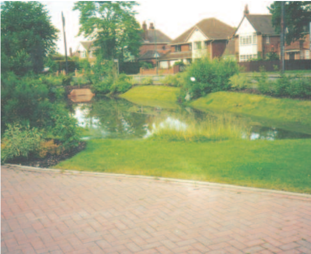
Detention Basin, Ipswich
